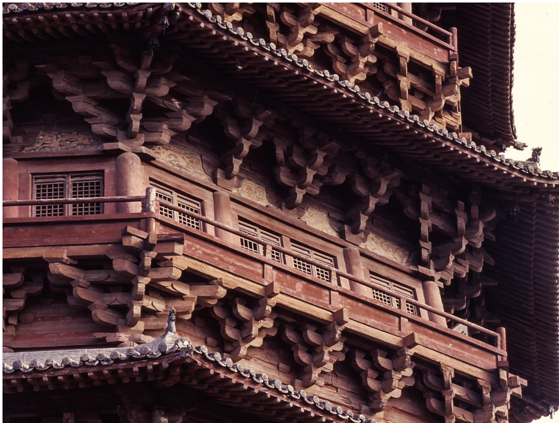
Figure 9. Corbelled Platform of the Wooden Pagoda of Ying County
