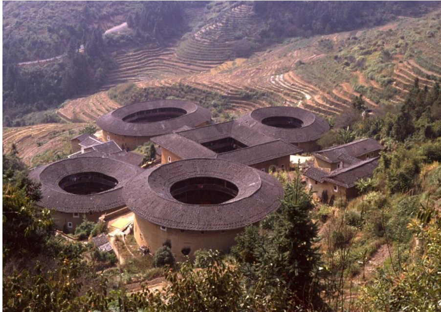
Figure 18. This village with five tulou (earthen buildings) are called Tianluokeng. Among them, two tulou were built during the Cultural Revolution (1966-1976). The reason was the same as that for building tulou in ancient times. At that time, people thought society was unstable, so they built tulou for self-protection.
