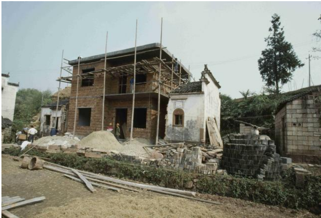
Figure 6. Traditional houses generally were not suitable for modern people's lifestyles. China also has had a severe shortage of wood. Therefore, farmers often demolished old houses and build new ones with bricks and concrete.
