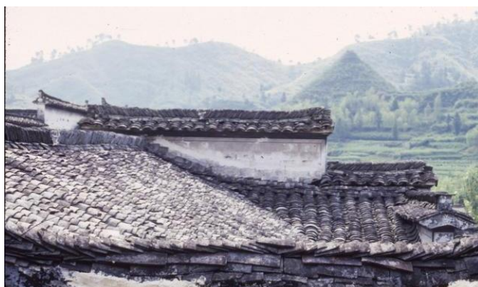
Figure 23. This is the roof of the houses surrounding a small courtyard in a traditional residential building in the southern Anhui region. The courtyard is very small, and all the rainwater from the roof flows into the courtyard.
