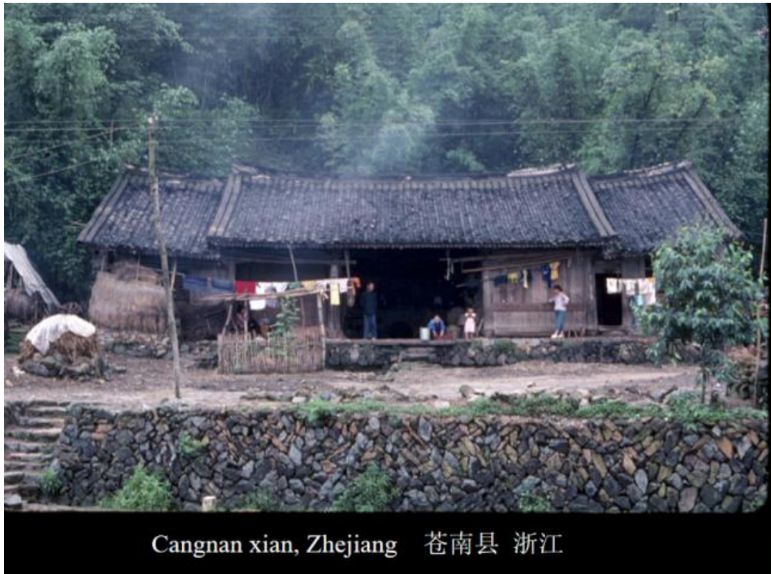
Figure 29. This is a residential house in Cangnan County, Zhejiang Province. The walls are made of wood. The two ends of the roof ridge are upturned, forming an elegant roof shape.
