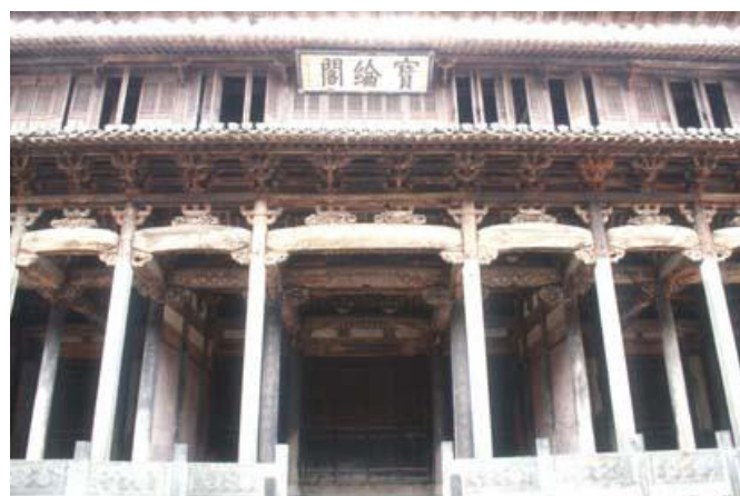
Figure 31. This is the exterior of the building in the last courtyard of Baolun Pavilion (an ancestral hall of a family). It is now a national cultural relics protection unit in China.
