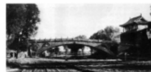
Fig. 1 Anji bridge, 1933 Zhuo county, Hebei province 40m Length 93.82 m (After Liang Sicheng, Liang Sicheng wenji , Beijing, 1982, p. 240)
