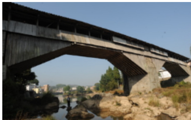
Qiancheng Bridge, Pingnan County, Fujian Province. Photo by Wang Qijun
